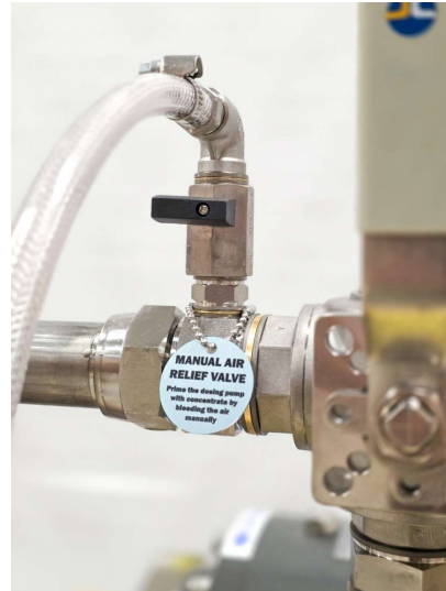
Manual Air Relief Valve with Dosing Return Valve
